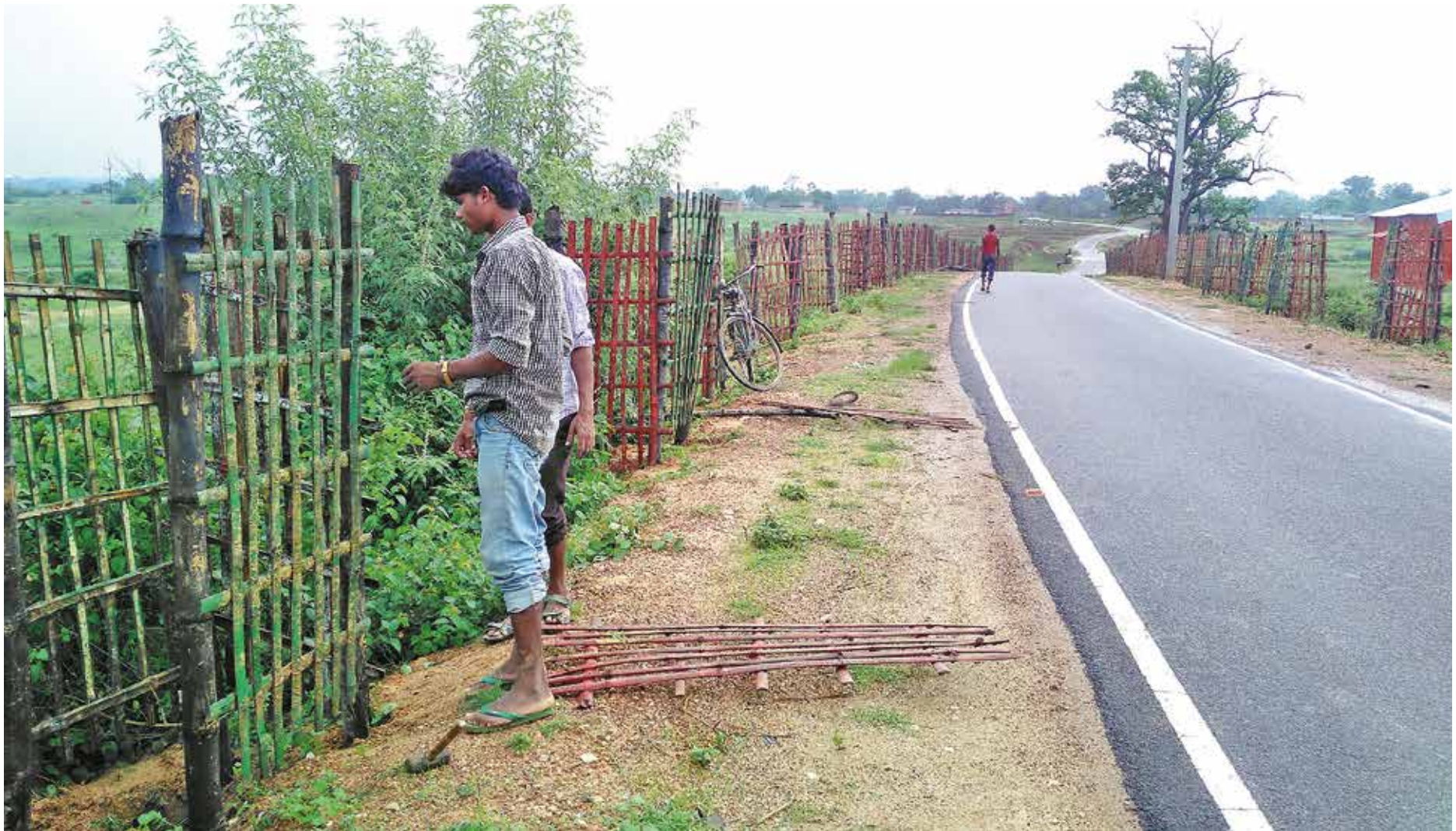
>> Erecting the gabiion structure for protecting tree plantation
