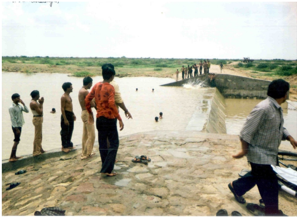
Check-dam: a unique water conservation method.
