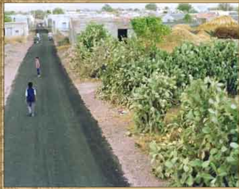
A Village Road Surfaced with Bitumen.
