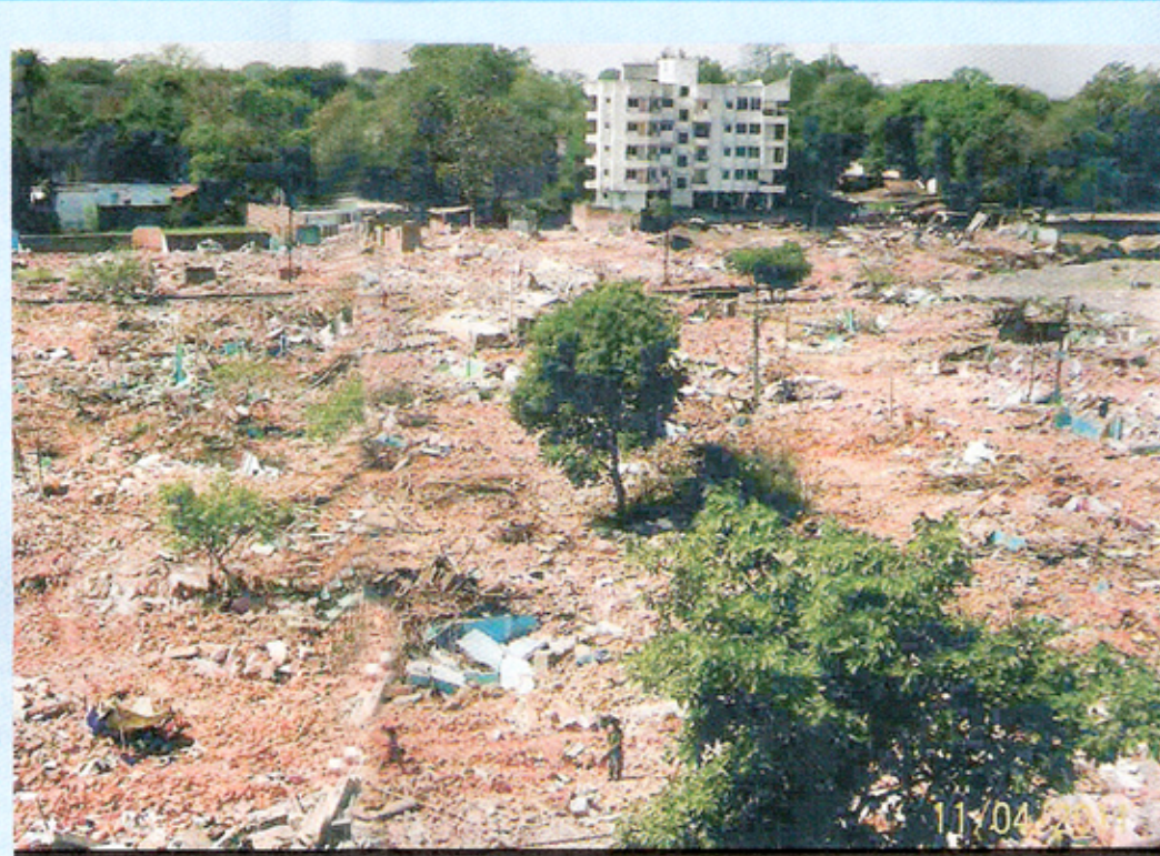
Islamnagar after demolition
